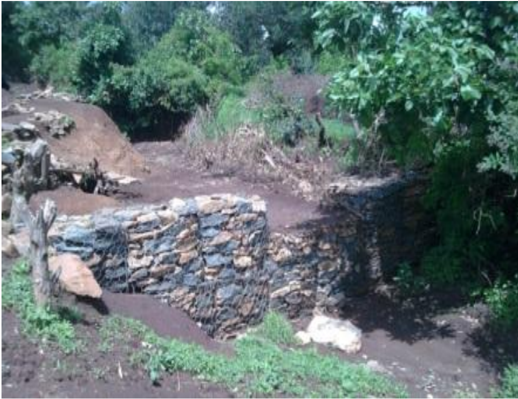
Checkdam- to rehabilitate gullies (Picture: Yinager)
