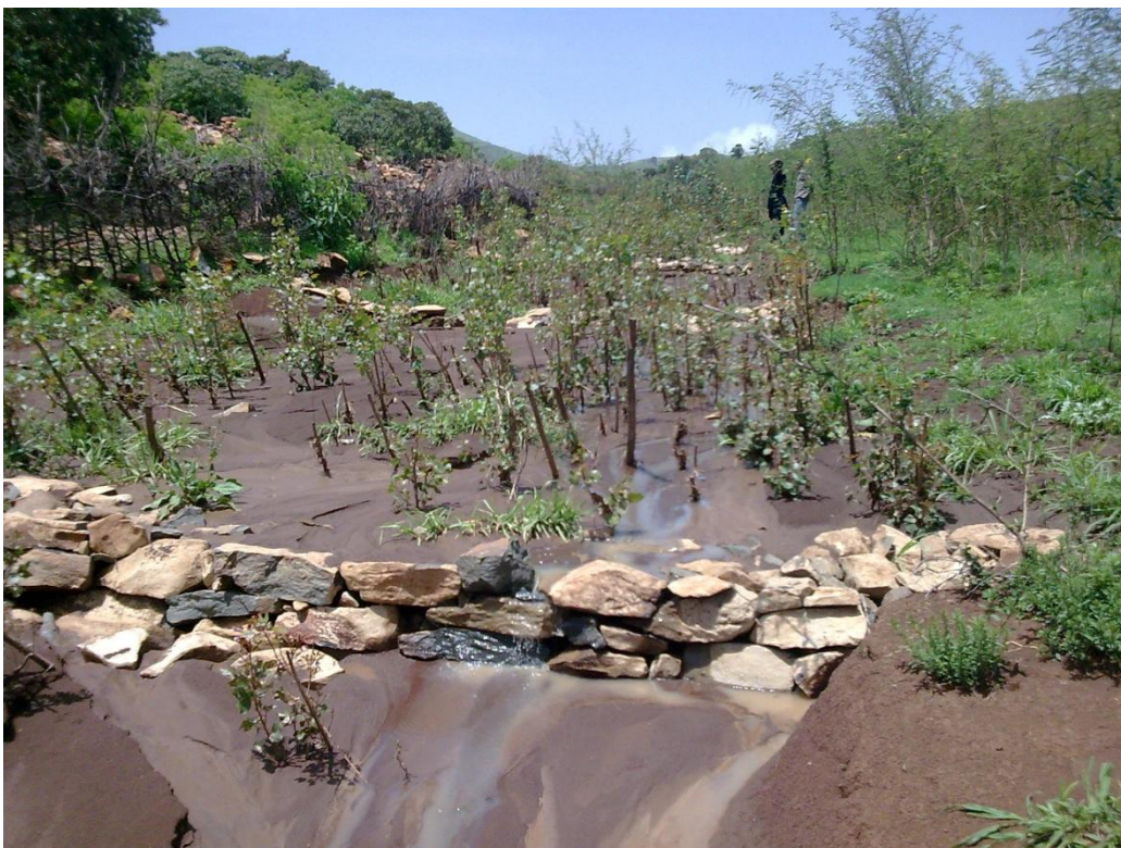
Stone terraces and plantations to rehabilitate a gully (Picture: Yinager)
